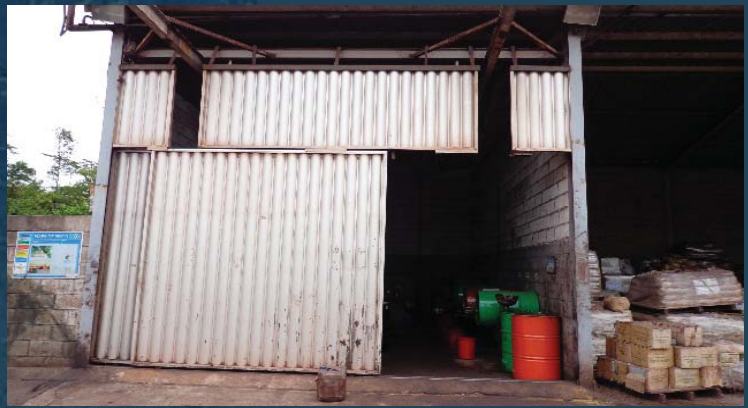
Samarco's old lube room was partially open, and access to the room was not controlled.
