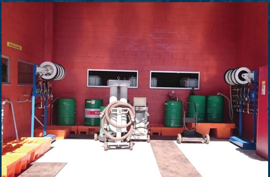
The lubricant receiving room is separate from the treatment rooms.
