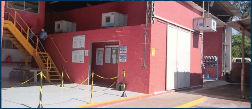
Access to the lube room is now controlled.
