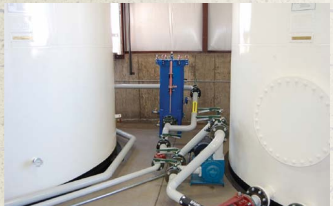
All incoming oils at Shoco Oil's bulk lube facility are pumped through individual filter canisters before entering bulk tanks.
