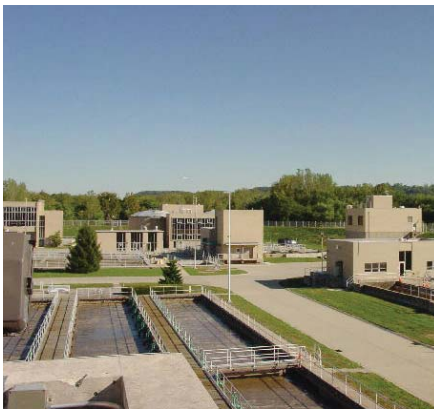
The Metropolitan Sewer District Wastewater Treatment Division operates seven major treatment plants and more than 100 smaller treatment facilities that process an average of 180 million gallons of raw sewage each day.
