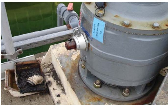
An oil sight glass with dirty oil (left) and clean oil (right)
