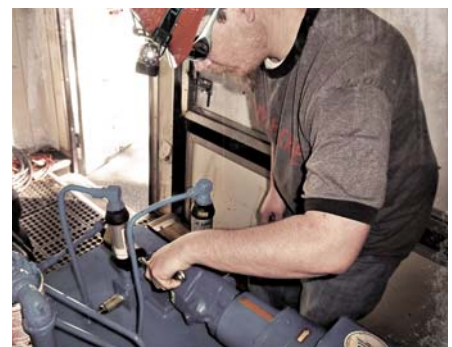
Knobs on hydraulic pumps and valves are often adjusted without any idea of the effects on the machine.
