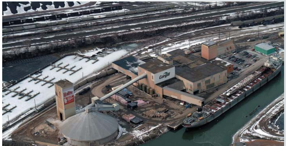
Cargill Deicing Technology's rock salt mine in Cleveland, Ohio, is 1,800 feet deep and extends approximately 4 miles under Lake Erie.
