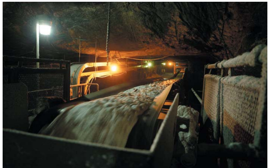
Salt is loaded onto a conveyor system for transfer to the milling operation, which crushes and screens the salt into a usable product before transporting it to the surface.
